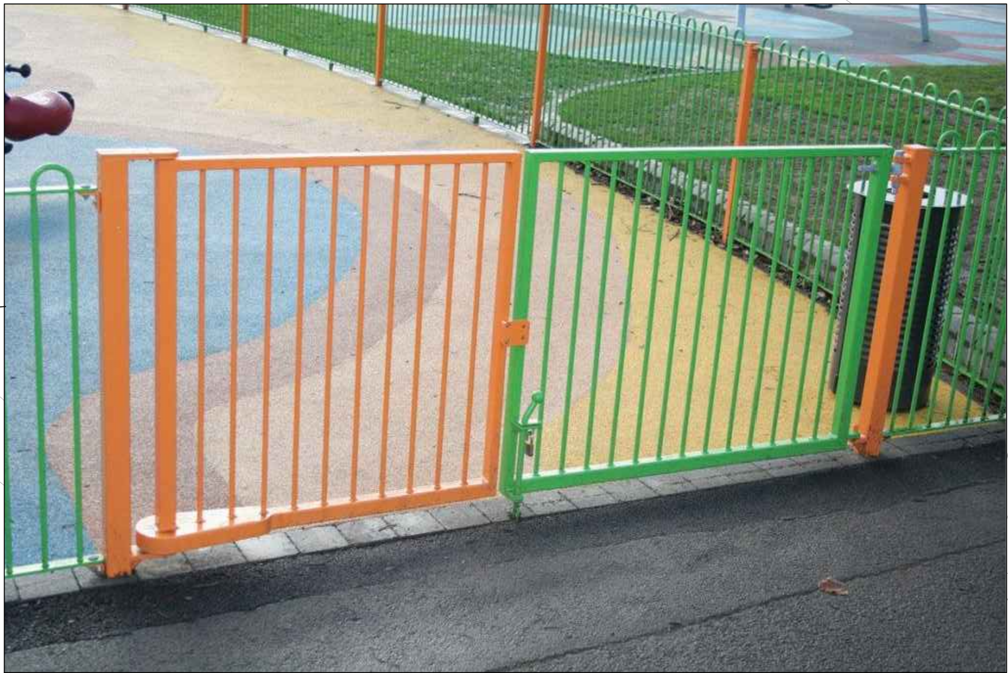
Combined Vehicle/Pedestrian gate
