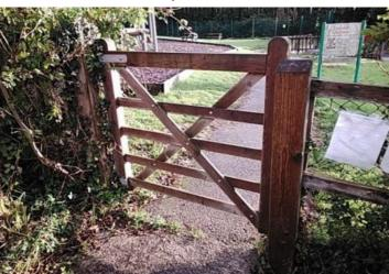
Finding: The gate is closing too quickly (less than 4 seconds)
