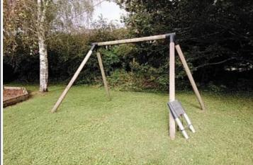
**Finding:** There is significant tree growth within the falling space of the unit
