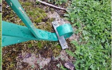
**Finding:** A number of ground anchor fixings are slightly loose
