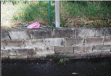
Finding: The retaining wall is damaged and some of the blocks are working loose
