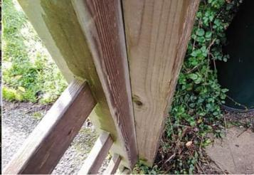
Action: Where possible a 12mm gap should be maintained on both sides or between the gate leafs
