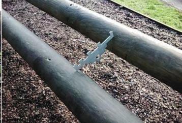
Finding: The item fails to meet the requirements of BS EN Action: Monitor - No remedial work recommended 1176 Part 1 4.2.7.2 for head and neck entrapment between the beams
