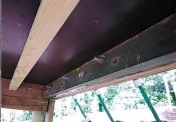
**Action:** Remove excess thread length and deburr or provide cap
