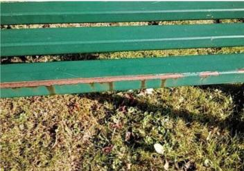
Finding: The paintwork on this item has been damaged or Action: Treat any rusting components and repaint worn exposing the metal underneath which is rusting
