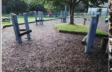
**Finding:** The depth of the loose fill surfacing is lower than the recommended depth specified in BS EN 1176; the free height of fall of the equipment is less than 2.0m and a minimum of 300mm depth should be provided (including an extra 100mm to allow for compaction and displacement as per BS EN 1176 Part 1 - Table 4)
