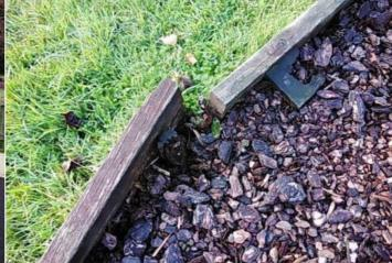
Finding: Parts of the bark pit edging are damaged / rotted / Action: Repair as required
