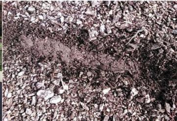
Finding: The depth of the loose fill surfacing throughout the Action: Top up loose fill surfacing to recommended levels bark pit area is lower than the recommended depth specified in BS EN 1176; the free height of fall of the equipment is less than 2.0m and a minimum of 300mm depth should be provided (including an extra 100mm to allow for compaction and displacement as per BS EN 1176 Part 1 - Table 4)
