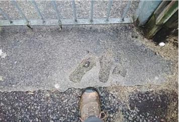
**Action:** Reinstate surrounding surfaces to level to remove the trip points
