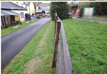
**Finding:** Most of the fence is either very loose in the ground **Action:** Repair as required to secure the fence or the posts have sheared at ground level. The fence is mostly unstable.
