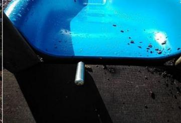
**Finding:** There is/are finger entrapment/s in the slide and the item fails to meet the requirements of BS EN 1176 Part 1
