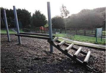
**Finding:** The item fails to meet the requirements of BS EN 1176 Part 1 4.2.7.2 for head and neck entrapment between the beam and post
