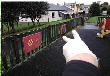
**Finding:** 4x timber posts have rotted and sheared and the fence is unstable
