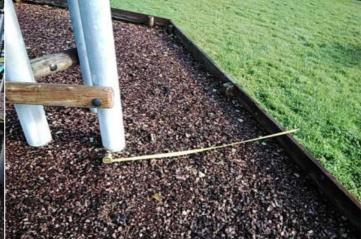
**Finding:** The edging forms a hard object within the falling space of the equipment in contravention of the requirements of BS EN 1176 Part 1
