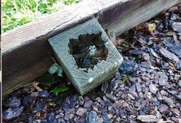
**Finding:** There is some evidence of rot in the timber bark pit **Action:** Monitor for any further deterioration and replace as edging
