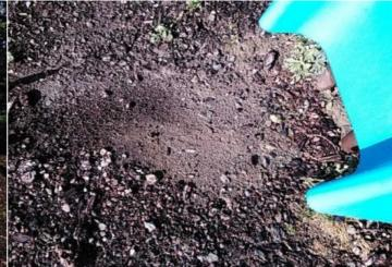
**Finding:** Bark mulch has been displaced from the end of the **Action:** Reinstate / top up mulch to ensure a minimum slide and the compacted, stoney sub-base is exposed depth of 300mm all around the unit
