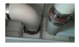
Asbestos Content: Contains (1) Chrysotile asbestos fibres.
