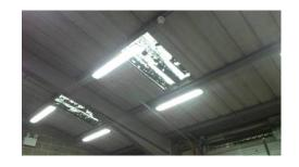
Asbestos Content: Strongly presumed to contain (1) Chrysotile asbestos fibres.
