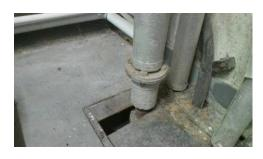
Asbestos Content: Contains (1) Chrysotile asbestos fibres.
