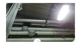
Asbestos Content: Contains (1) Chrysotile asbestos fibres.
