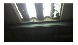
Asbestos Content: Strongly presumed to contain (1) Chrysotile asbestos fibres.
