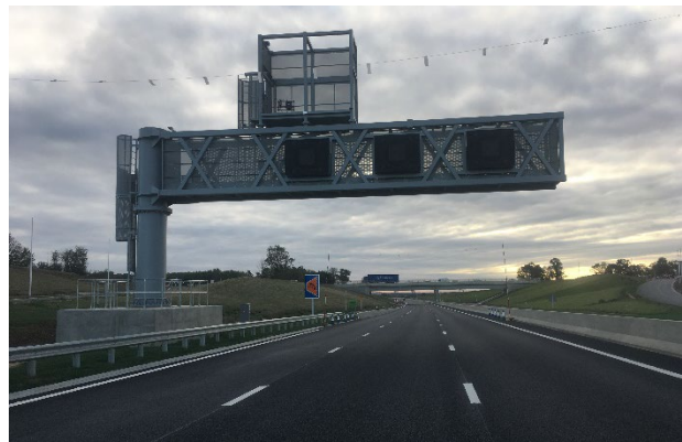
Super-span Cantilever Gantry (during A14 construction)
