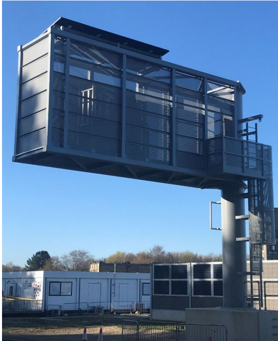
Cantilever Gantry (rear) illustrating depth of structure and protected maintenance access provision
