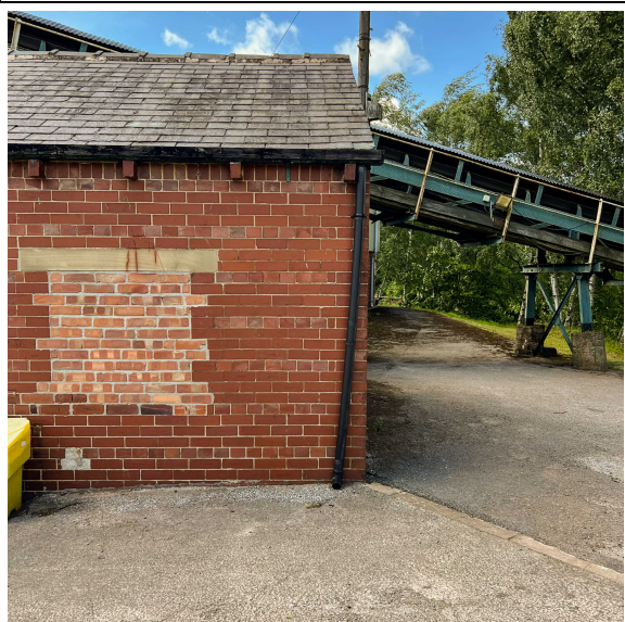
Control room: Front rainwater goods are still the old timber gutters and a poorly fixed plastic downpipe.
