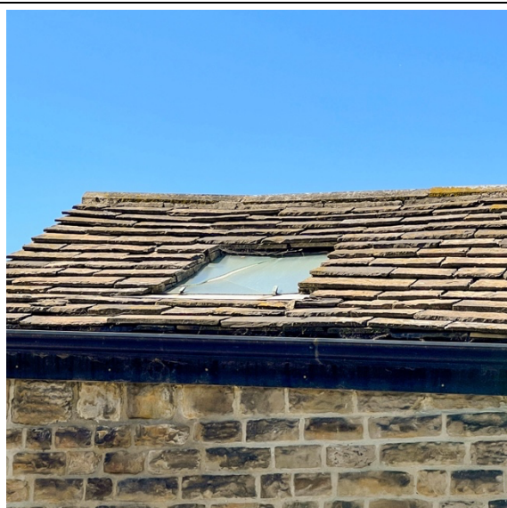
Roof: South side, Rooflight badly damaged
