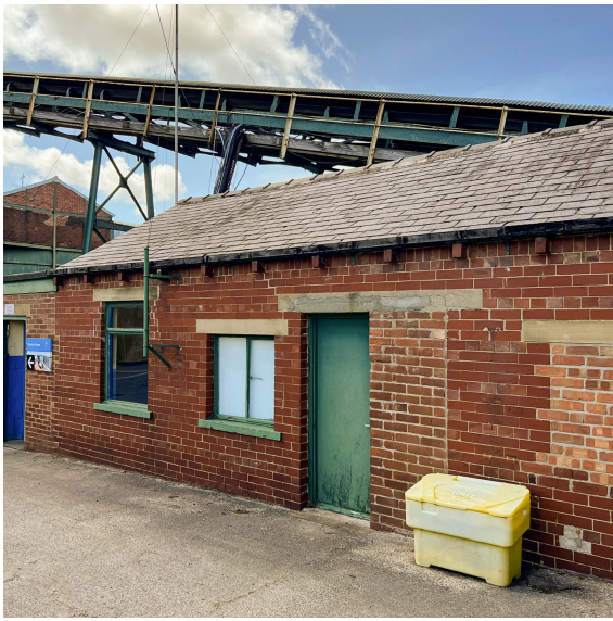
Control room: Access door in poor condition
