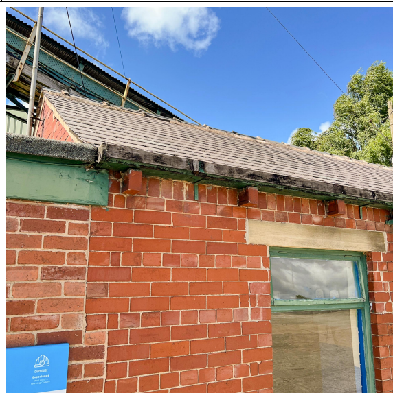
Control room: Front rainwater goods are still the old timber gutters and a poorly fixed plastic downpipe.
