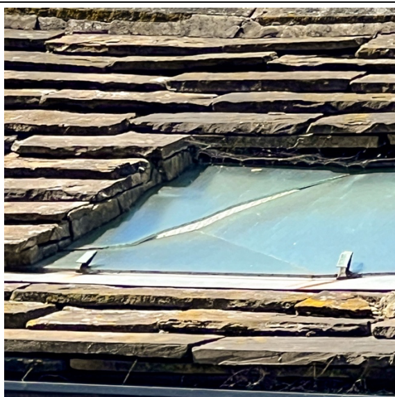
Roof: South side, Rooflight badly damaged
