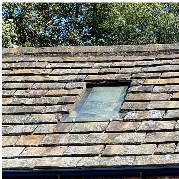
Roof: North side crudely detailed roof light
