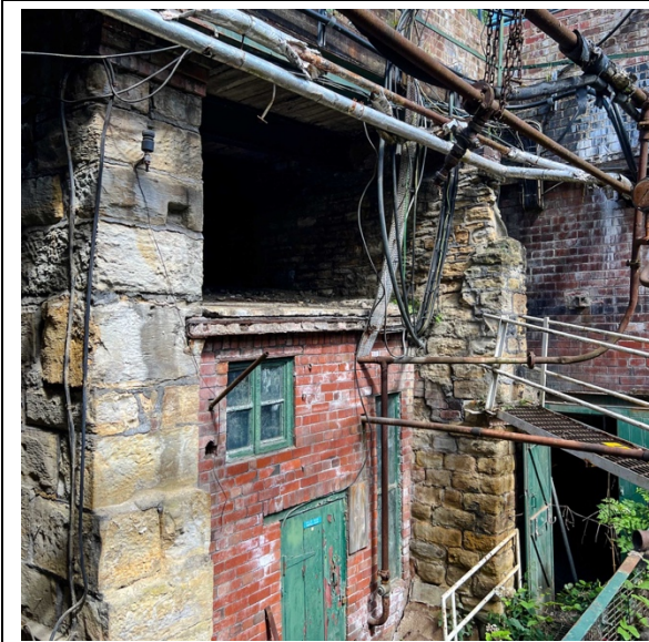
Lancashire boiler - Switch room general view
