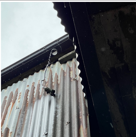
Screens building by metal stairs – gutter missing a down pipe and soaks the base of the stairs
