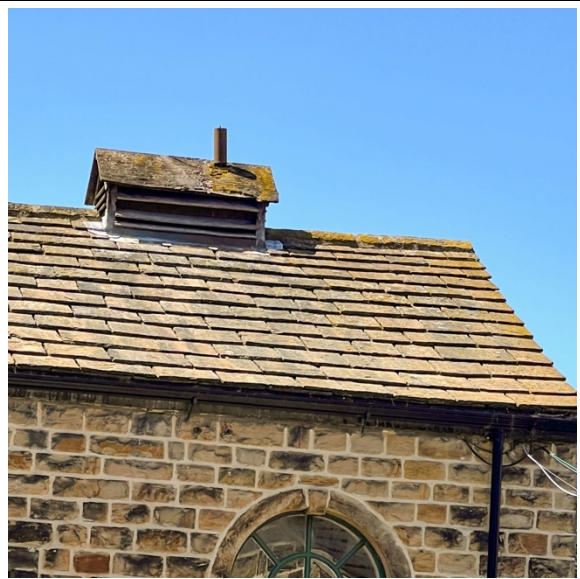
Roof: General view of south side
