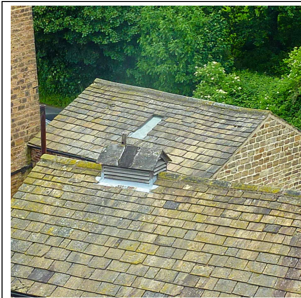
Roof: General views from the North
