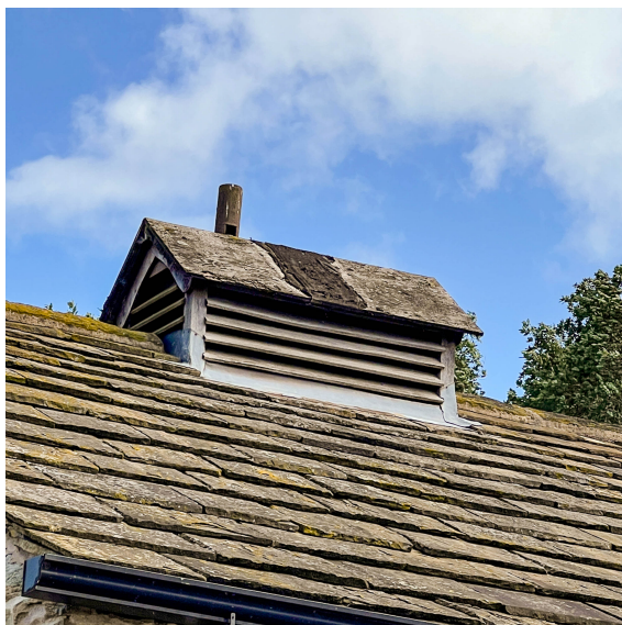
Roof: Ridge dormer has lost its covering leaving just decaying plywood
