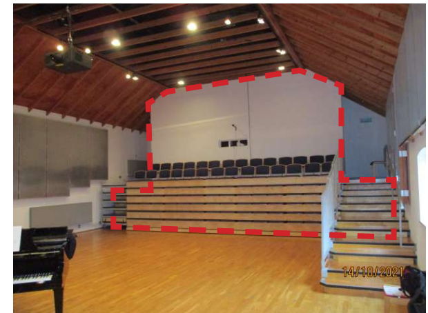
Photos of the existing Room. Red dotted line denotes the zone of demolition to remove the existing projection booth along with the sound and light lobbies
