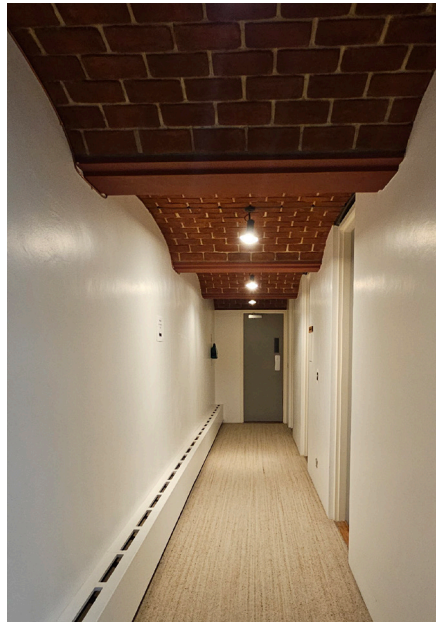
Photos showing the vaulted brick soffits of the concrete floor slabs
