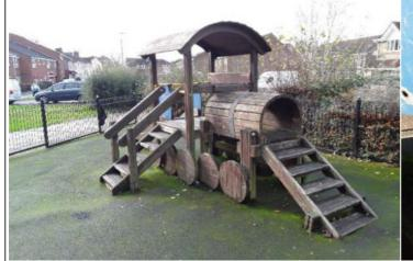
**Finding:** There is/are finger entrapment/s in the slide start section and the item fails to meet the requirements of BS EN 1176 Part 1 4.2.7.6 Entrapment of fingers
