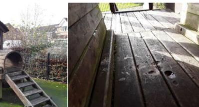
Finding: There is some evidence of fire damage to the item Action: Monitor for any further deterioration and repair as required
