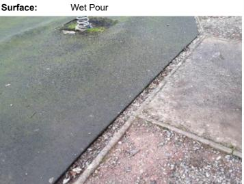
**Finding:** There are significant gaps (over 30mm) between the surface and the edging or between the joints in the surface; these are large enough for a small foot to enter
