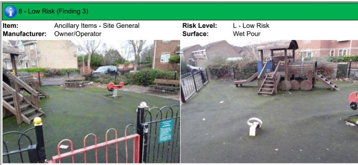
Finding: There is algae, silt or moss growth on the surface Action: Clean and treat appropriately resulting in slippery conditions
