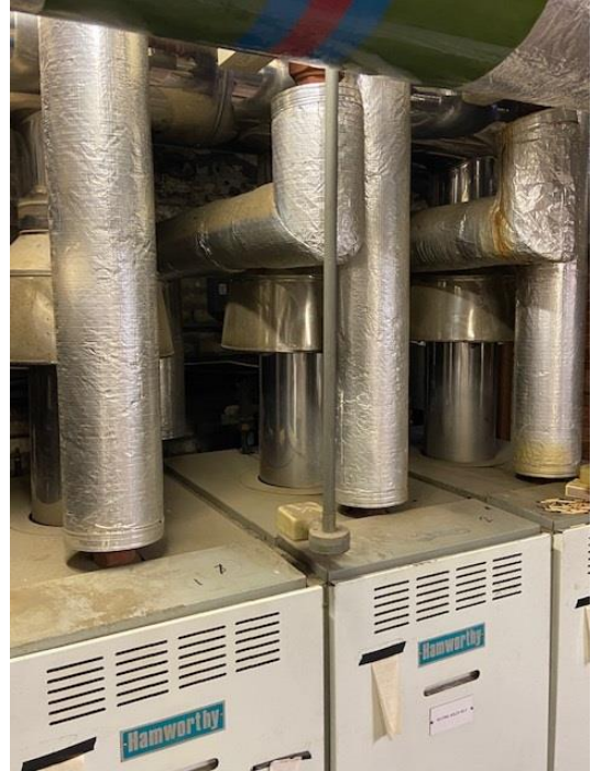
Existing Heating Flue System
