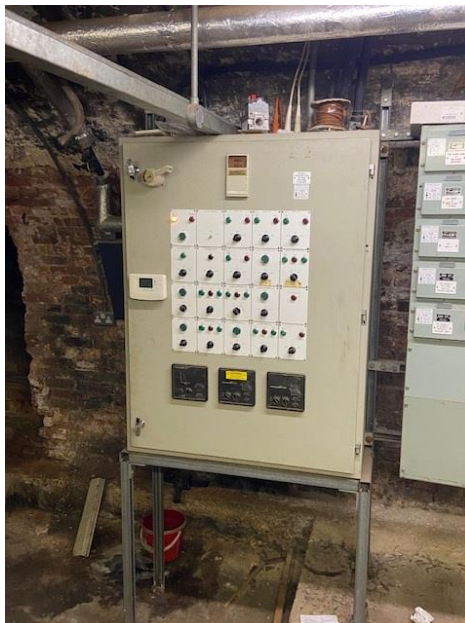
Existing Heating Control System
