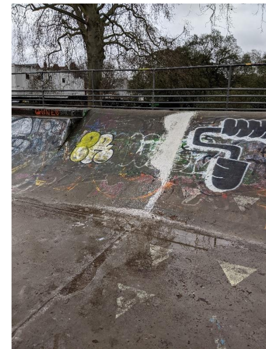
Figure 9 - Typical mirror crack in 2012 Concrete skim over top of units (white material is a DIY infill from local skateboarders)
