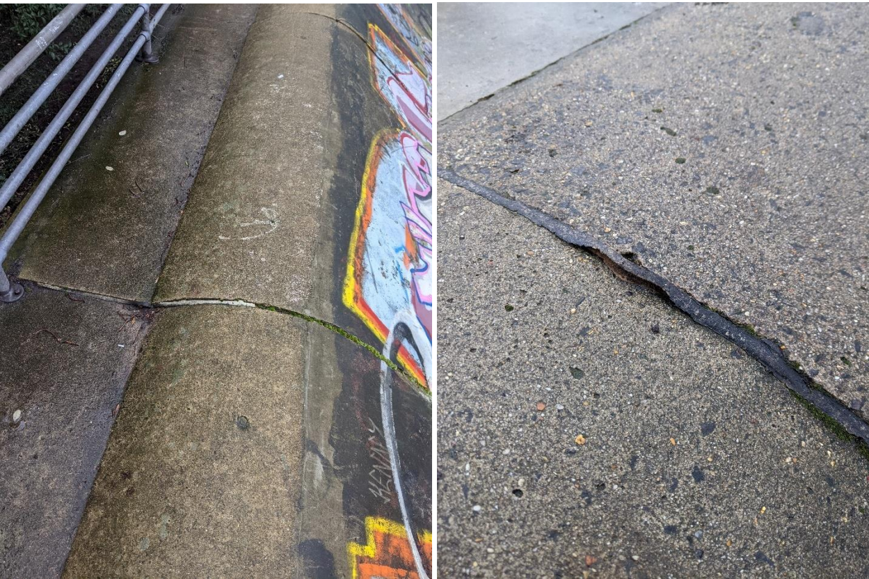
Figure 11 - Areas of gasket strips between units. Left: Partially removed sections with moss growth in between Right: compressed strips bulging out
