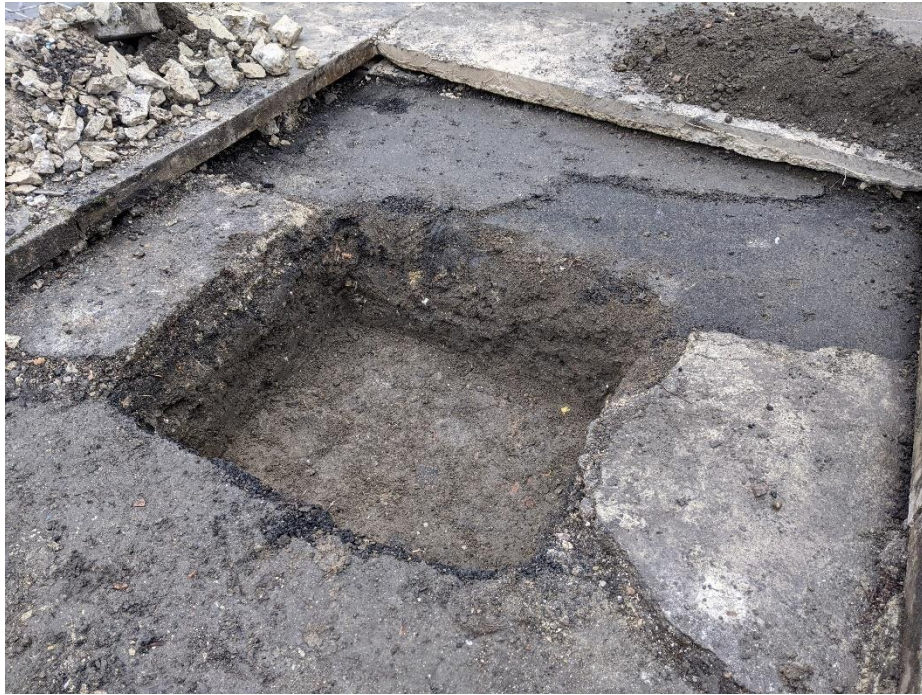
Figure 7 - Exposed trial pit and slab junction at northern end of skatepark. Existing tarmac on topsoil visible at top of picture with nominal mass concrete pads in foreground
