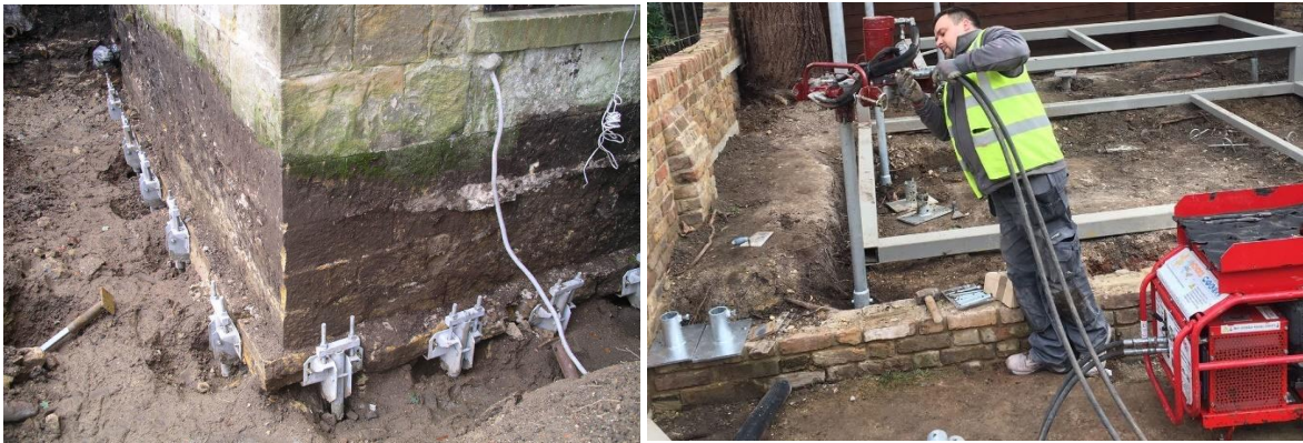
Figure 13 – left: Screw-pile underpinning installed onto subsiding masonry to external corner of residential property Right: Typical manual installation of helical screw-pile installation
