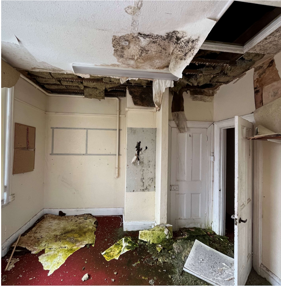
image00229 - WH First Floor North
