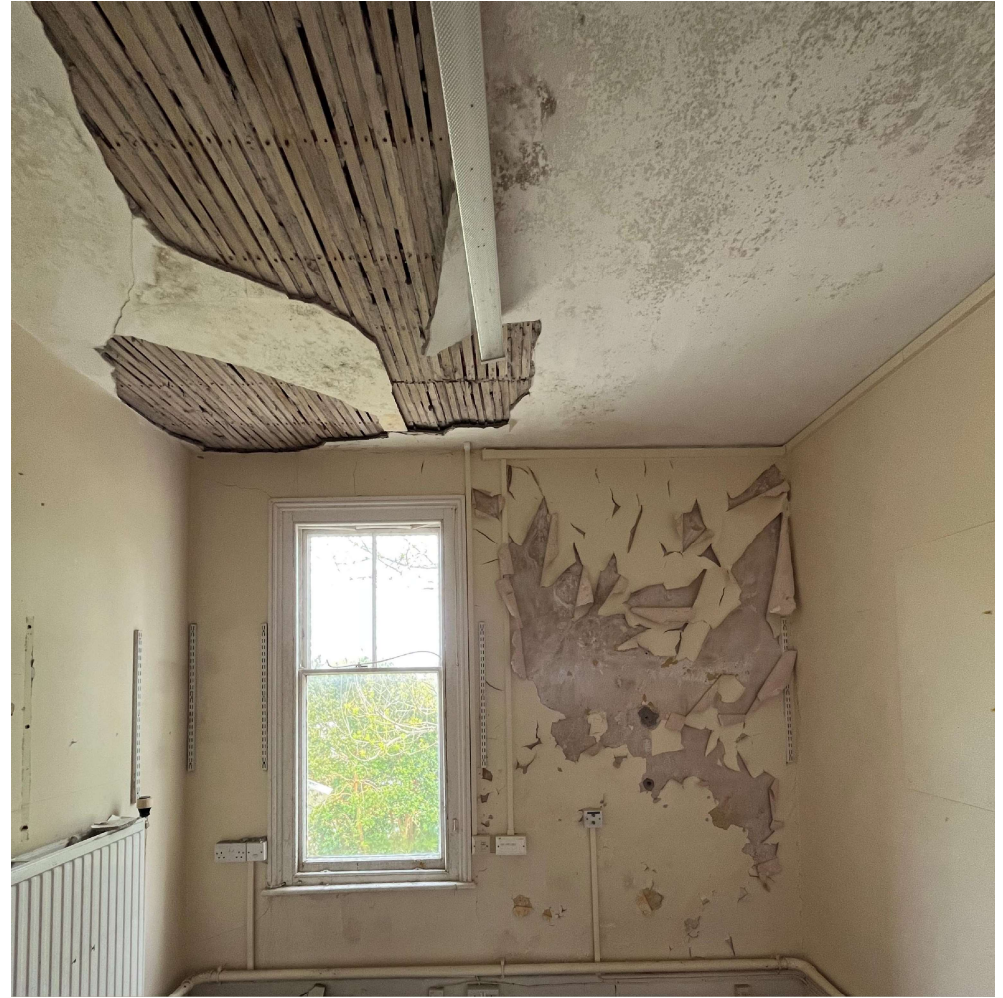
image00237 - WH First Floor North
