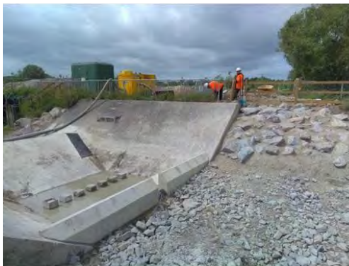
Images of recessed eel tiles at Burnt Mill gauging weir and testing of mounted and recessed tiles at Lydney.
