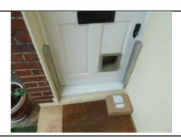
A barrier will include all fixings and all necessary modifications to existing door and surroundings and installation of required permanent fittings and frames, all necessary reinstatement, durable silicone based sealant around the frame, matching the existing and to the required protection height, and around sills to seal all gaps.
