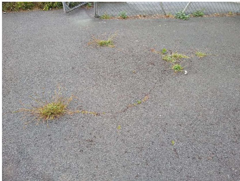
Typical Cracked Surface
