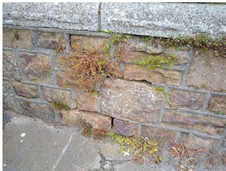
Typical Condition of Granite stone wall
