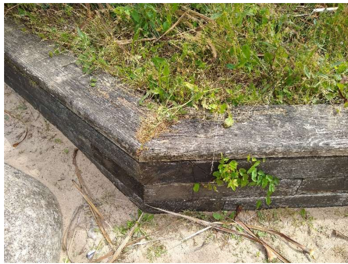
Sleeper Retaining wall to planting
