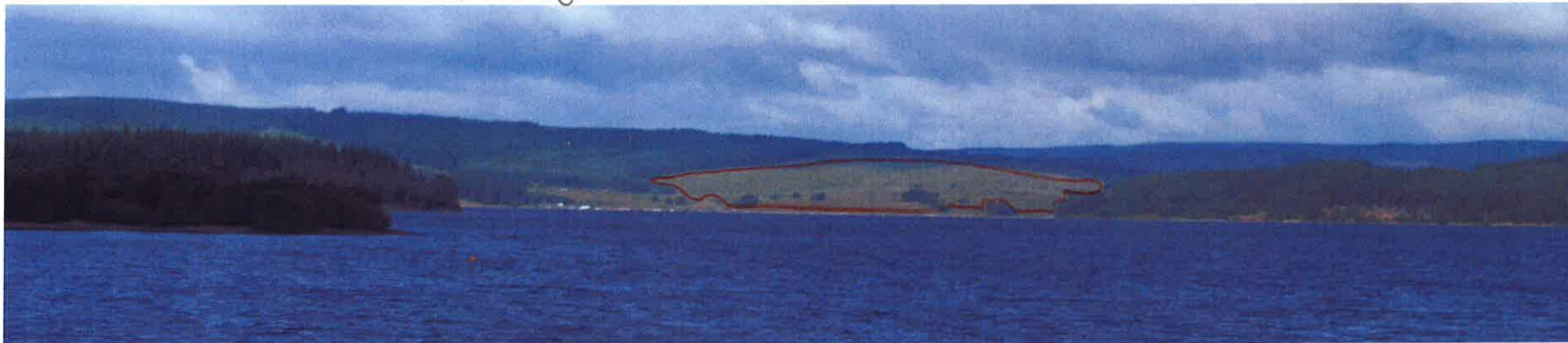
View from Kielder Dam to Rushy Knowe
