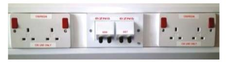
6. The faceplates shall be wired such that minimal cable is coiled immediately behind it. However, sufficient spare cable shall be provided to enable at least 3 re-terminations at the UP. Care must be exercised to ensure that cable bend limitations are not exceeded.
