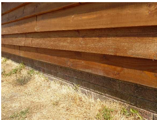
Fig 5: Proposed cladding over brick plinth
