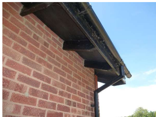
Fig. 6: Proposed eaves detail (as existing pavilion)
